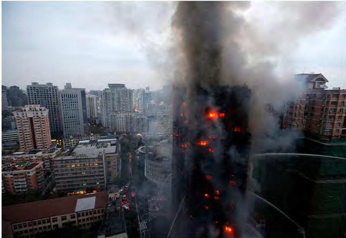
Firefighters try to extinguish a fire at a 28-story apartment building in Shanghai, Monday Nov. 15th, 2010. The blaze killed 53, and sent over 70 to hospitals. Preliminary
