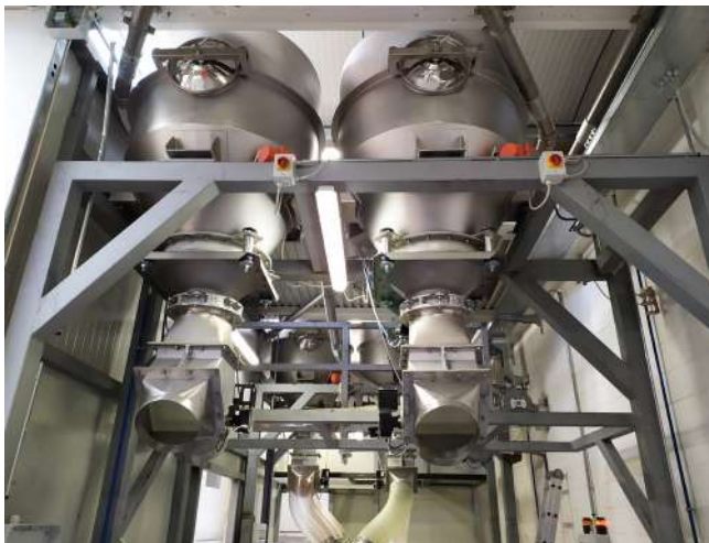
4 hoppers to receive the product on a mixer for milk, sugar and cocoa transport.
