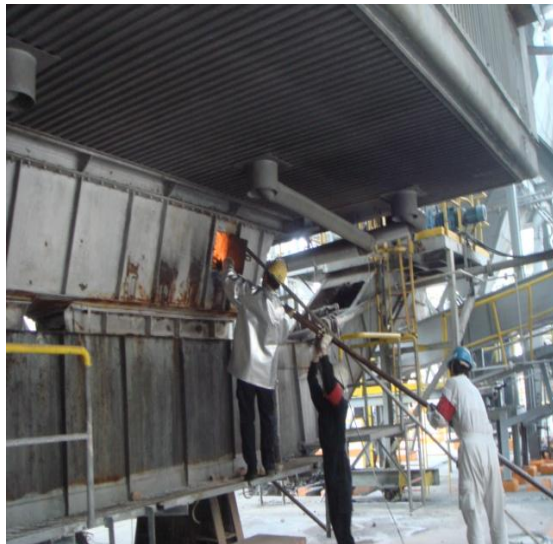
置入鍋爐結塊內 Insert the tube into clinker
