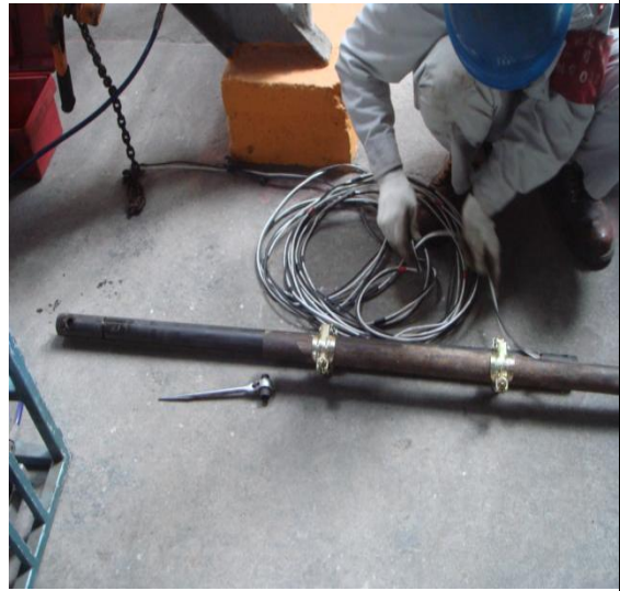
準備高壓管並扣緊延伸管 Prepare Tube and fix with an extend-tube
